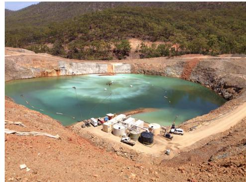
> Hydrotalcite treatment in progress - subsurface spraying
