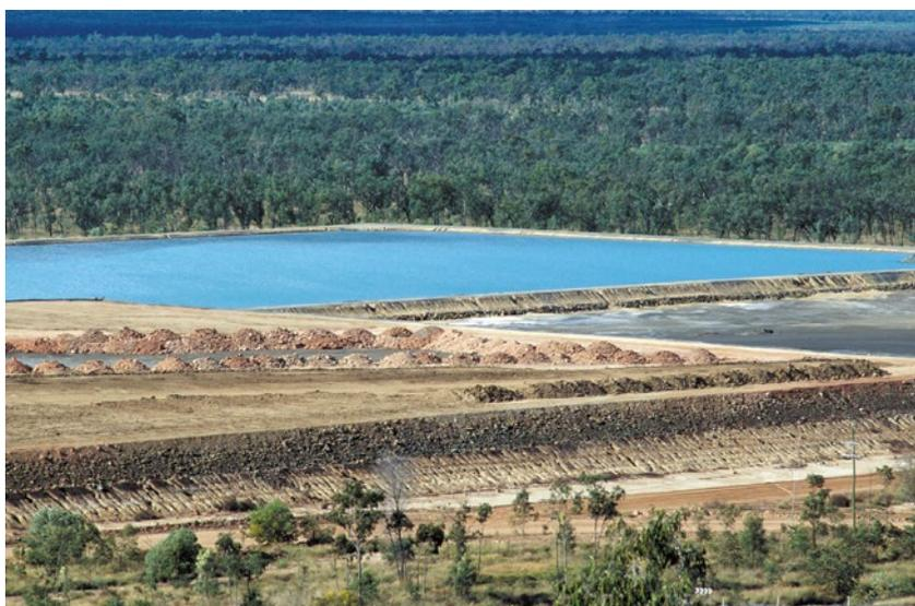
Mining wastewater, such as in these tailing ponds, can contain a variety of contaminants that can be difficult to remove.
